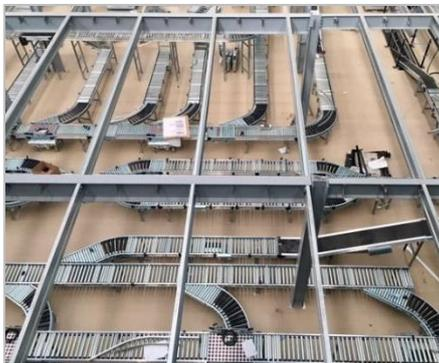
The conveyors that will transport stock totes and packages around the warehouse have been built and we are now in the early stages of physical testing. This process will initially test the delivery of totes from one point to another.
