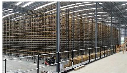
The assembly of the pallet racking for bulk storage is nearing completion. The racking, featured in the image above, comprises 35 aisles and will cover the majority of the warehouse floor space.
