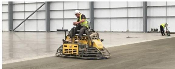
It is important that the floor is exactly flat. As manual picking will take place at up to 18 metres high, the slightest discrepancy at ground level could introduce significant deviation at that height.
