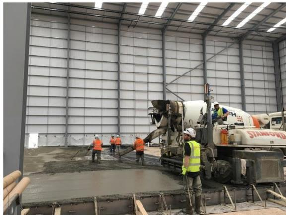
The concrete was poured in sections and then levelled by a topping spreader. Once each batch had set, the top was then levelled and smoothed by a machine that glides across the surface like a small hovercraft.
