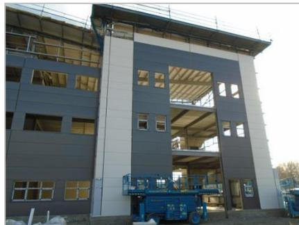
Following the completion of the roof and exterior walls, the warehouse is now weather-proof and this has allowed internal construction work to start.
