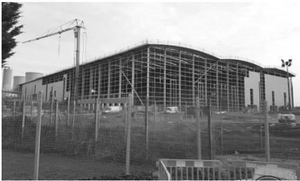
Following the completion of the main framework of the building, exterior cladding is currently being applied to create the outer walls and a roof.
