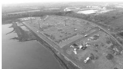
During January, steel uprights will be erected that will form the framework of the new warehouse. A waterproof shell will be built around the frame by the end of February that will then allow internal construction work to take place.
